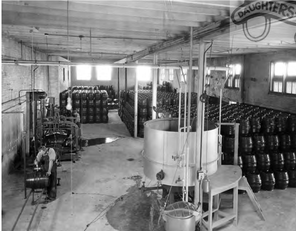
Filling and sealing beer kegs at Fisher Brewing Company. (Used by permission, Utah State Historical Society)
